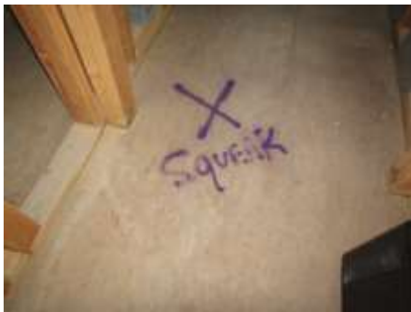
Secure loose and squeaking third level sub floor
