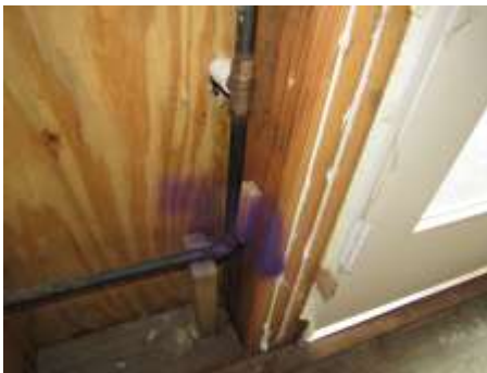
Secure gas pipe to balcony
