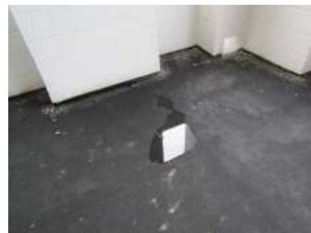
Ponding water on fourth level balcony
