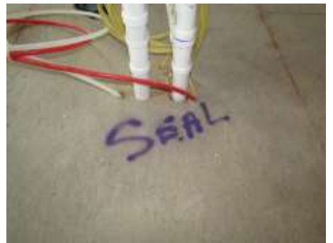
Seal voids at kitchen water, electric and drain pipes
