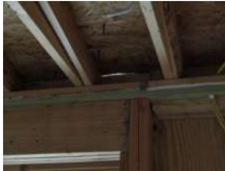
Daylight around edges of fourth level roof
