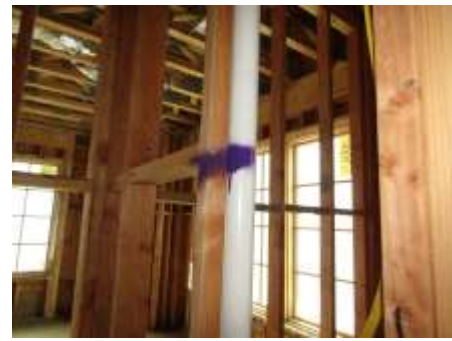
Strap loose PVC drain piping
