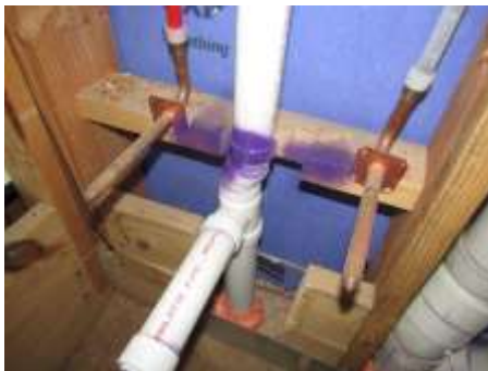
Strap loose PVC drain piping
