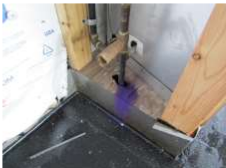
Seal gas piping at balcony fireplace
