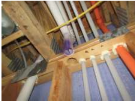
PVC pipe securing drain above
