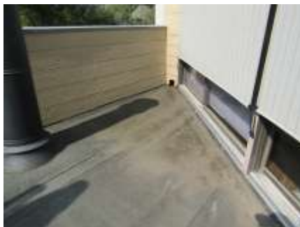
Area of ponding water and excess sealant at door and glazing
