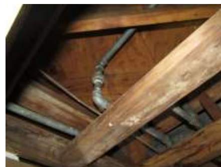
Galvanized steel water piping
