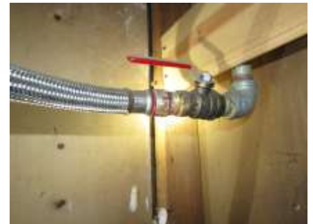
Corrosion on fitting
