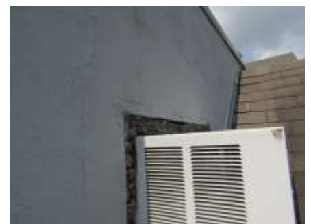
Poor sealant around third level window unit
