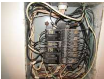
Hot right feed wire and on breaker at guest quarters panel
