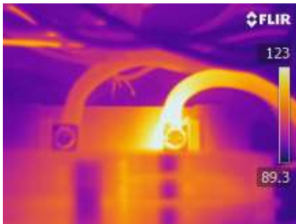
Heat image of 123 degrees on sub panel right feed leg
