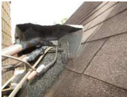
Void at roof jack for HVAC piping
