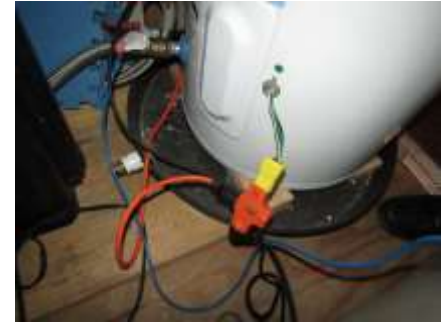
Improper electric connection for upper guest quarters water heater
