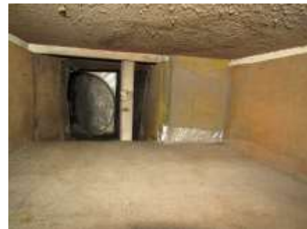
Clean and seal first level return chase
