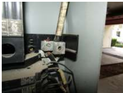
Corrosion on buss and connector
