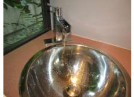
Weak water pressure at powder lavatory
