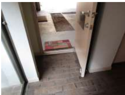
Door must be self-closing
