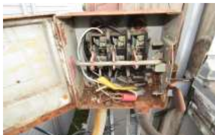
Corrosion on buss and connector
