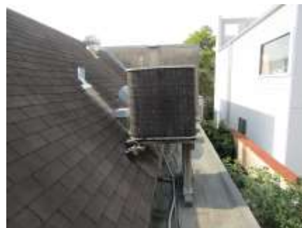
Abandoned A/C and wood frame
