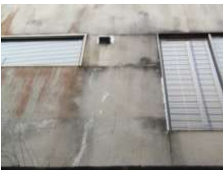
Stained stucco with cracks
