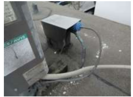
Missing insulation on guest quarters A/C
