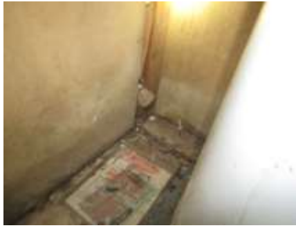
Stains in north water heater closet
