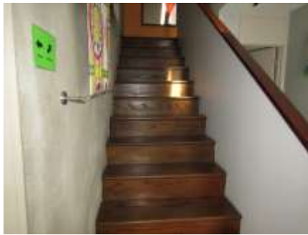
No grippable handrail
