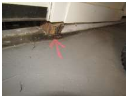
Damaged wood in garage storage door
