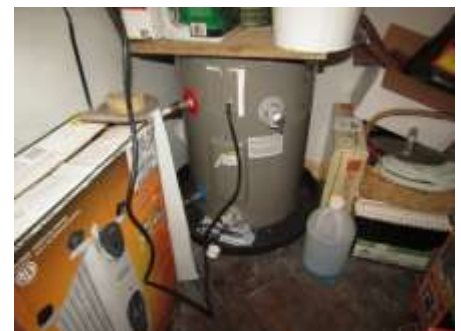
Secure cord and no drain off pan and safety valve at guest quarters
