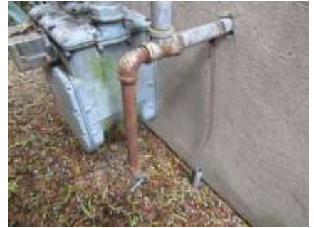
Rusted piping and old gas stop for previous pool heater
