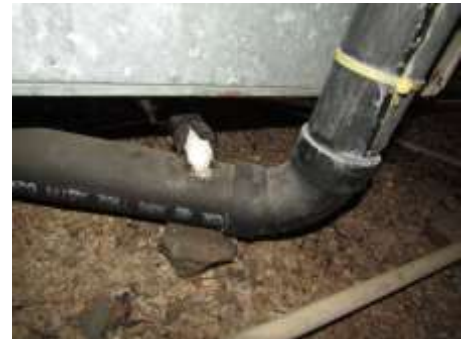
Primary drain in drain waste
