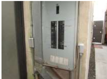
Poor labeling of breakers
