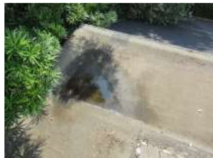
Ponding water on roof
