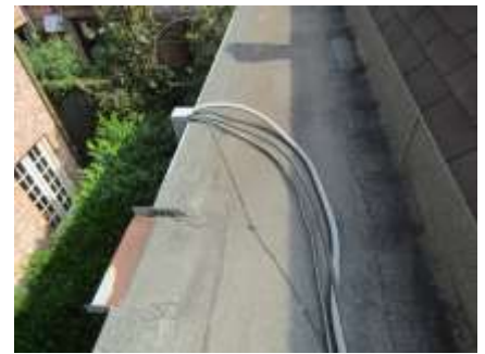
No protection of refrigerant line and conduit
