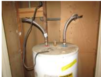
Loose wire and connection and missing disconnect
