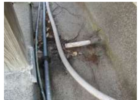
East HVAC emergency drain terminates on roof
