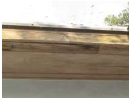
Loose and stained fascia and soffit
