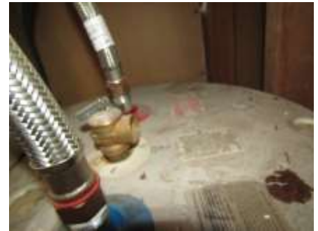
Missing safety valve drain
