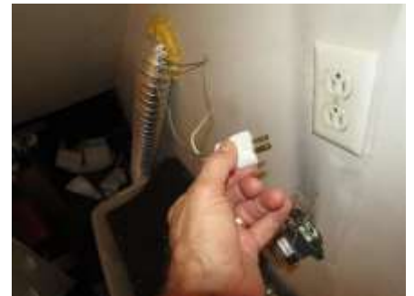
Poor wiring of guest quarters bathroom light and fan
