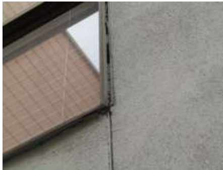
Poor sealant at windows
