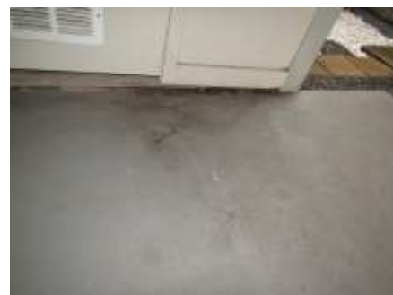
Water stains on concrete slab in garage
