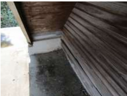
Loose, dry and unpainted wood
