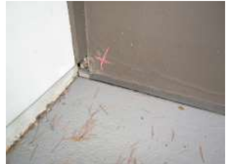
Damaged base of garage door panel
