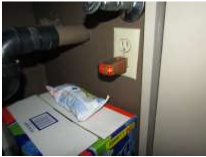
Not GFCI under wet bar
