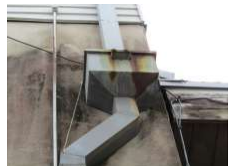
Stained stucco/plaster and rusted roof gutter box
