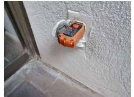
Exterior outlets not GFCI
