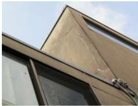
Stucco cracks and repairs
