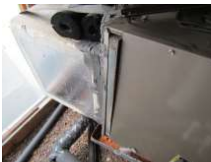
Remove old filter off east HVAC unit
