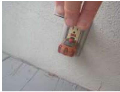
Front exterior GFCI not responding
