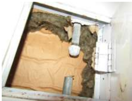
Gas stop valve removed at breakfast room fireplace
