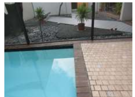
Heave and deflection of pool beam and tile
