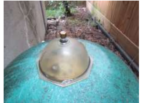
Missing gauge on dome
