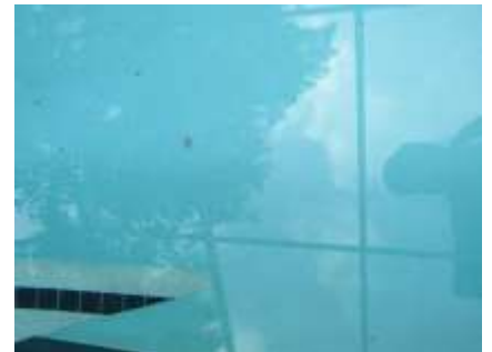
Crack in pool plaster
