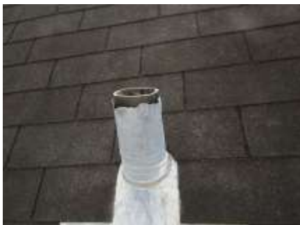
Damaged lead roof jack
