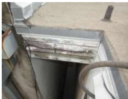
Worn and damaged wood
