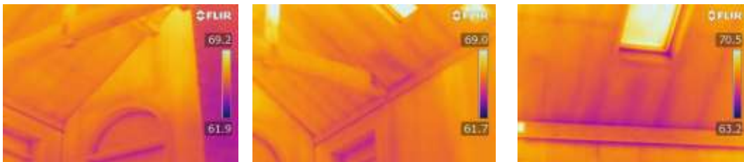
No anomalies on ceiling and walls of family room
