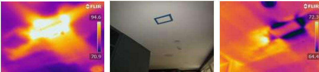
Image of covered air register with drywall in north hallway
