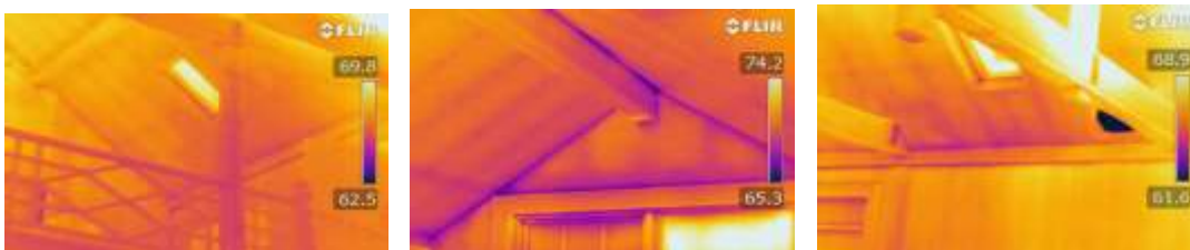
No anomalies on ceiling and walls in family room
