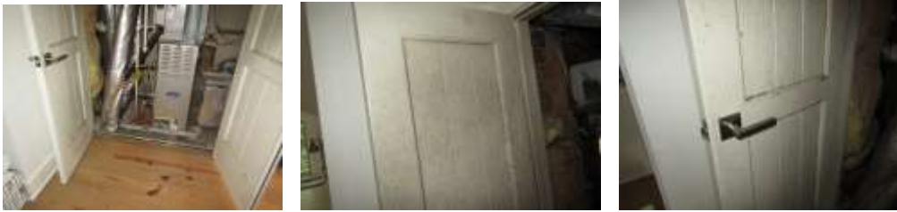
Black organic matter inside of double doors in 2 nd south bedroom HVAC
