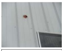
Missing light for junction box on south wall
