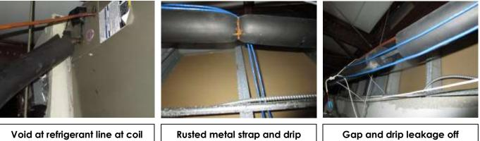
usted metal strap and drip leak off insulation on refrigerant line
