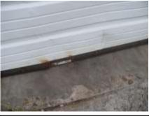
Rusted and damaged bay door panel
