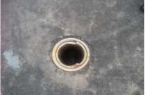
Clearstream Aerobic septic system installation. (D) Excessive dirt, ants, etc. on equipment and pumps at front of office building. Cap missing on suspect tank at rear northeast of building.
