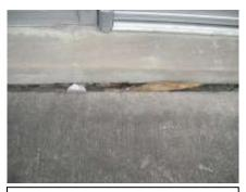
Damaged wood expansion joints
