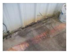
Stained metal panels from gutter leaks
