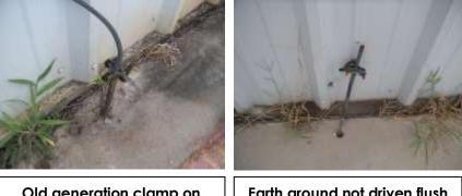
Old generation clamp on earth rod Earth ground not driven flush to grade and old clamp
