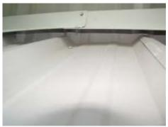
Missing foam inserts for wall panels at A/C unit enclosures
