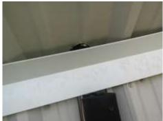
Seal voids at A/C refrigerant lines in wall panels
