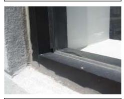
Voids at upper window metal frames and gasket
