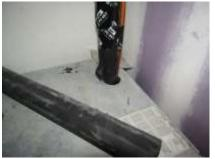
Air leaks at refrigerant lines in coil cabinets
