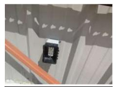
Plastic cover missing off front electrical outlet
