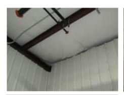
Water damaged insulation at rear northeast corner of warehouse
