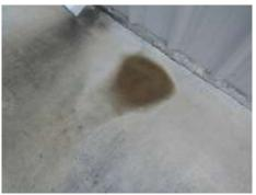
Stained flatwork from gutter leakage
