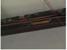
HVAC refrigerant line gaps from missing insulation
