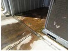
Excessive algae and water from clogged east A/C drain basin
