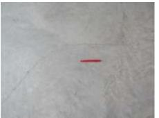
Concrete temperature cracks in second level concrete
