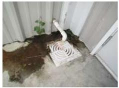
Wet flatwork from poor A/C drain termination
