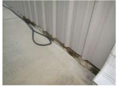
Water leakage along west side building and wall panel
