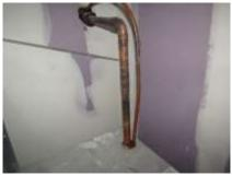
Second level suction/refrigerant line not insulated and sealed at cabinet
