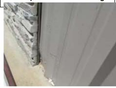
Seal voids at front east stone and wall panel
