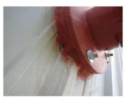
Poor sealant at fire sprinkler valves in wall panel siding
