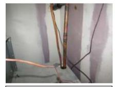
Missing insulation on second level west office refrigerant line
