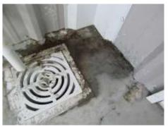
Water leakage off west side A/C drain
