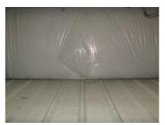
Bubble in insulation from water and roof leak
