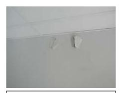
Drywall damages in second level wall
