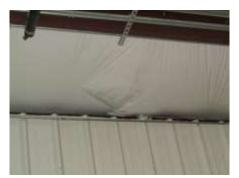
Damaged insulation under east warehouse roof from water leakage
