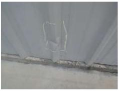
Damaged west side wall panel
