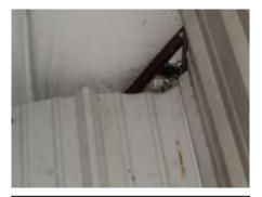
Void at west side wall panel and roof
