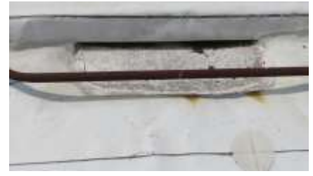
Narrow south drain scupper
