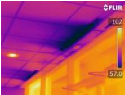
Quality air supply out of slotted air registers
