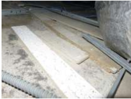
Stained acoustic tiles and mold/mildew
