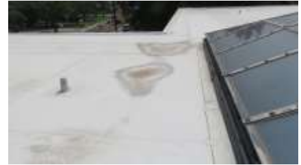
Dark area from ponding water
