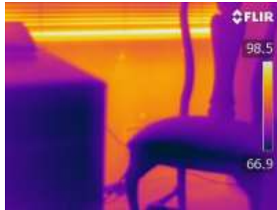
No anomalies under 1 st level windows
