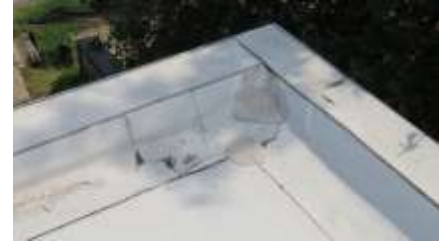
Repairs to roof
