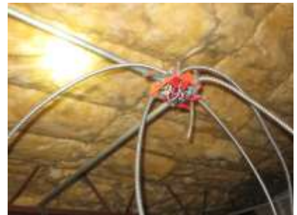
Exposed wires
