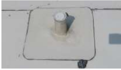
Capped drain waste vent on roof
