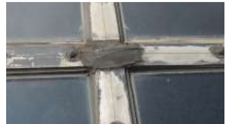
Tar sealant on skylight
