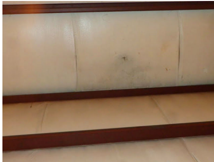
Stained insulation under roof
