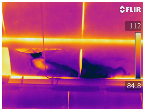
Images of moisture from active roof leakages on insulation
