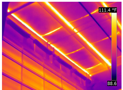
No anomalies under roof and on insulation
