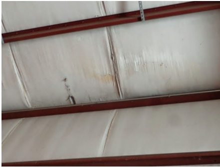
Stained insulation under roof
