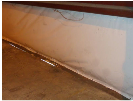
Daylight along lower outer edges
